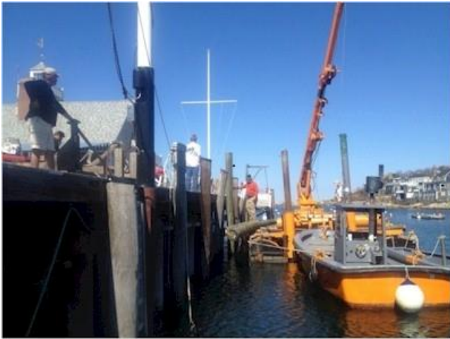
Tiger & crew(Braely & Myles) installing new pilings
